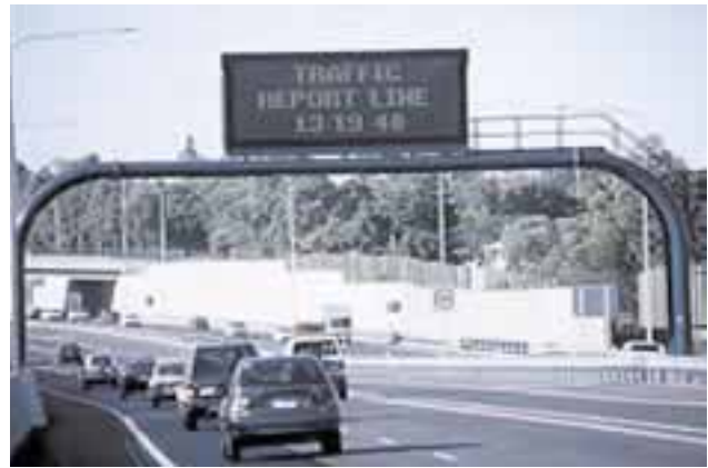
Variable message sign used to convey road safety messages and traffic management information.
